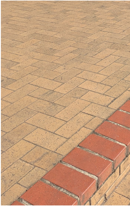
Existing brick paving
