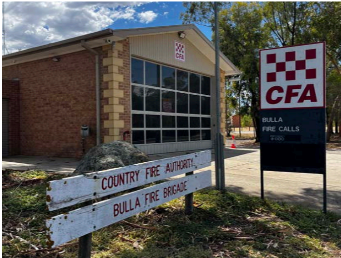
Figure 09: Bulla CFA Fire Station
