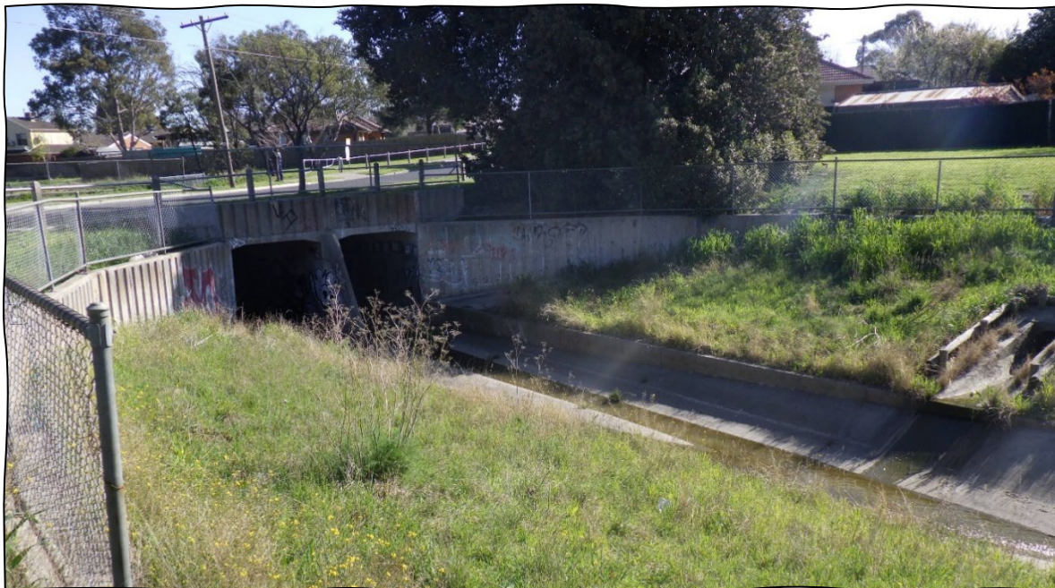
Figure 7 - Concrete channelled section of Merlynston Creek south of Hepburn Street, Dallas
