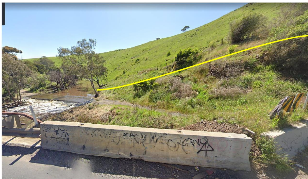
Figure 1 Holden Ford and approach road and extent of HO29 (yellow line)
